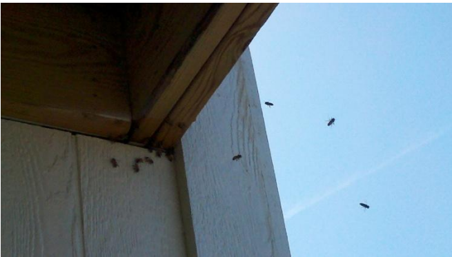
Honey bees entering wall void between 2 nd and 3 rd floors of an apartment building
