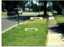
Damaged and Undamaged
